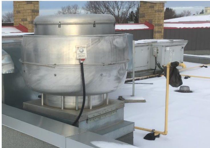
Photo 17: Large kitchen exhaust fan (left), MUA unit is seen on right in background
