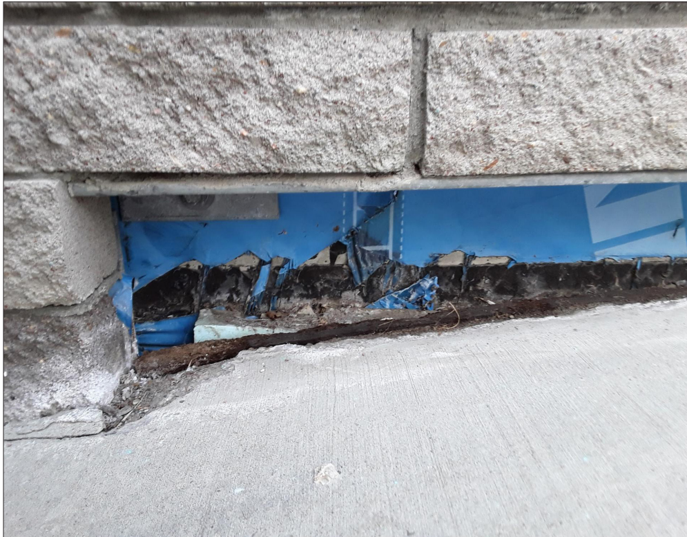
Image: Air/Vapour Membrane
