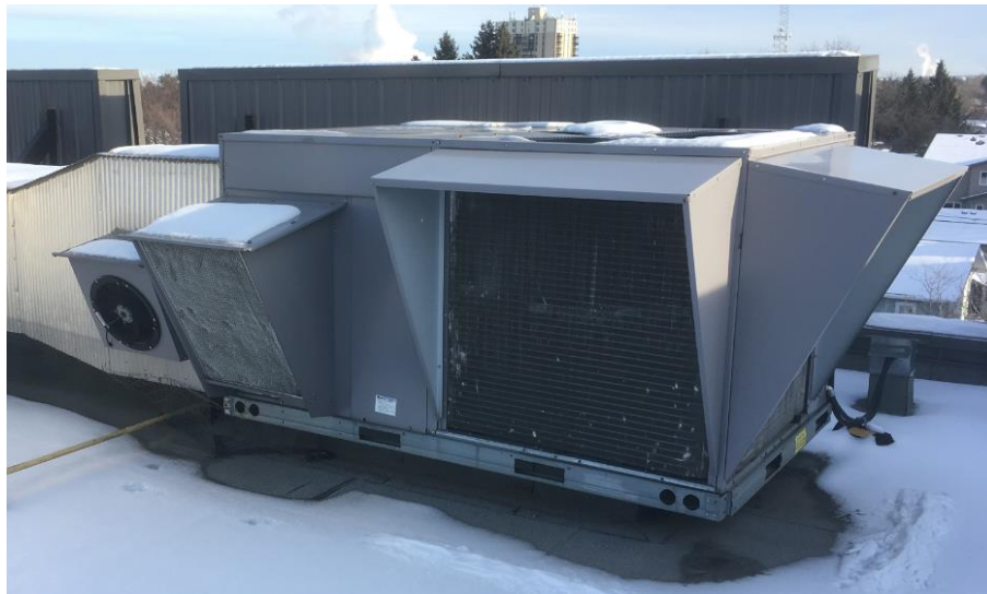
Photo 6: RTU-15 manufactured in 2009, located on Phase 2 roof
