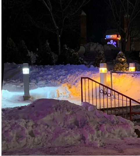
Exterior Bollards (note the two illumination colours – HPS and Metal Halide or Colour Corrected HPS)
