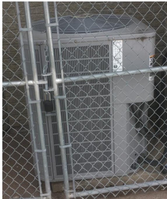
Photo 8: Air conditioning condenser
