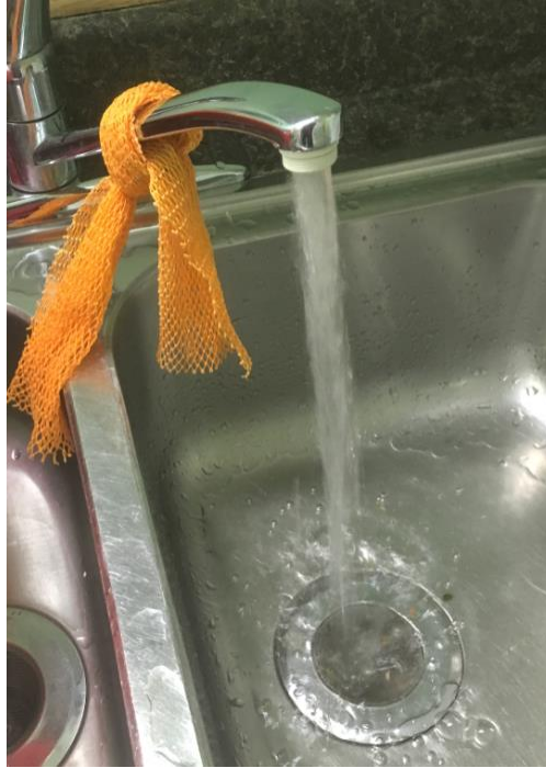
Photo 22: La Cité faucet with no aerator installed
