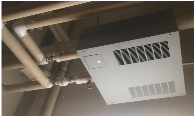
Photo 9: Forced-flow hydronic heater in stairwell
