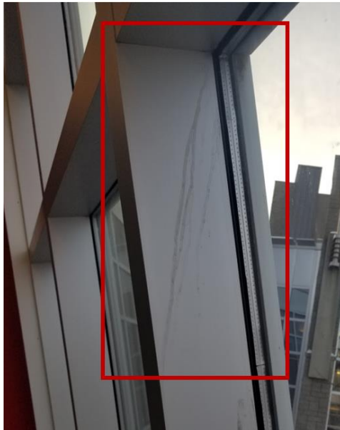
Photo 4: Possible window seal failure
