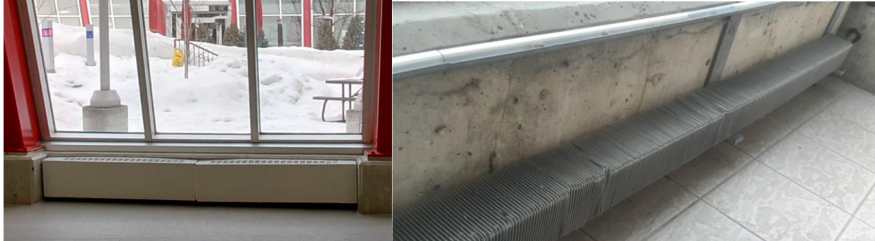
Photo 11: Perimeter radiant hydronic baseboard heater at base of windows (left), shown with cover removed (right)
