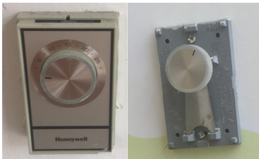
Photo 20: La Cité vestibule non-programmable thermostats
