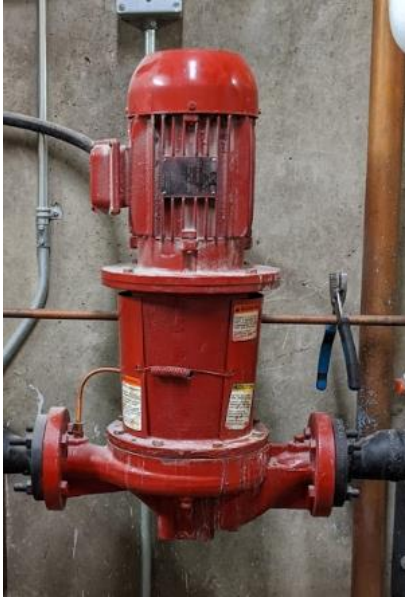
Photo 16: Boiler water circulation pump
