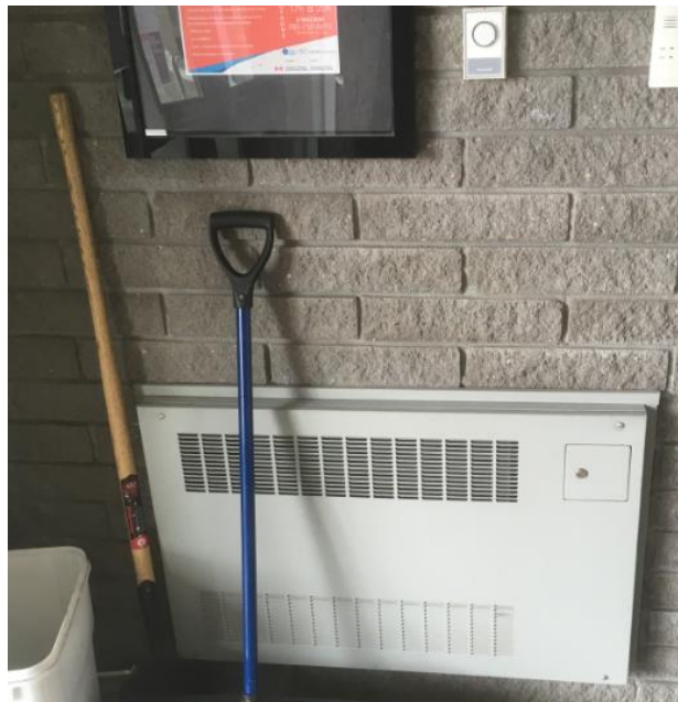
Photo 10: Entryway hydronic radiant heater, with manual thermostat above
