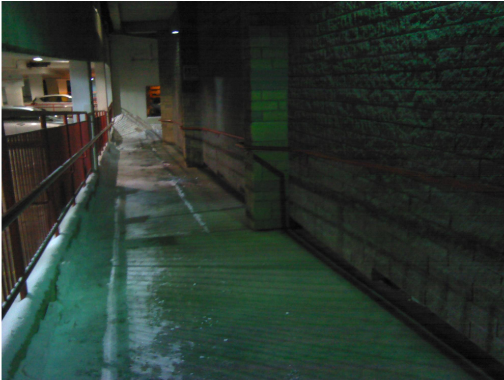
Images: Parkade to Building Transition, and Resulting Heat Loss
