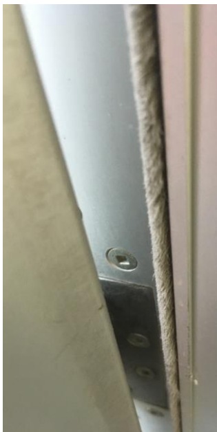
Photo 2: Door seal detail
